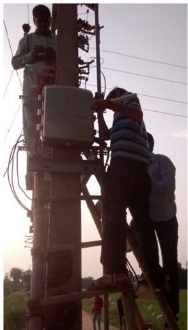
Figure 19 - Images from the installation of Smart meters for grid-connected households
