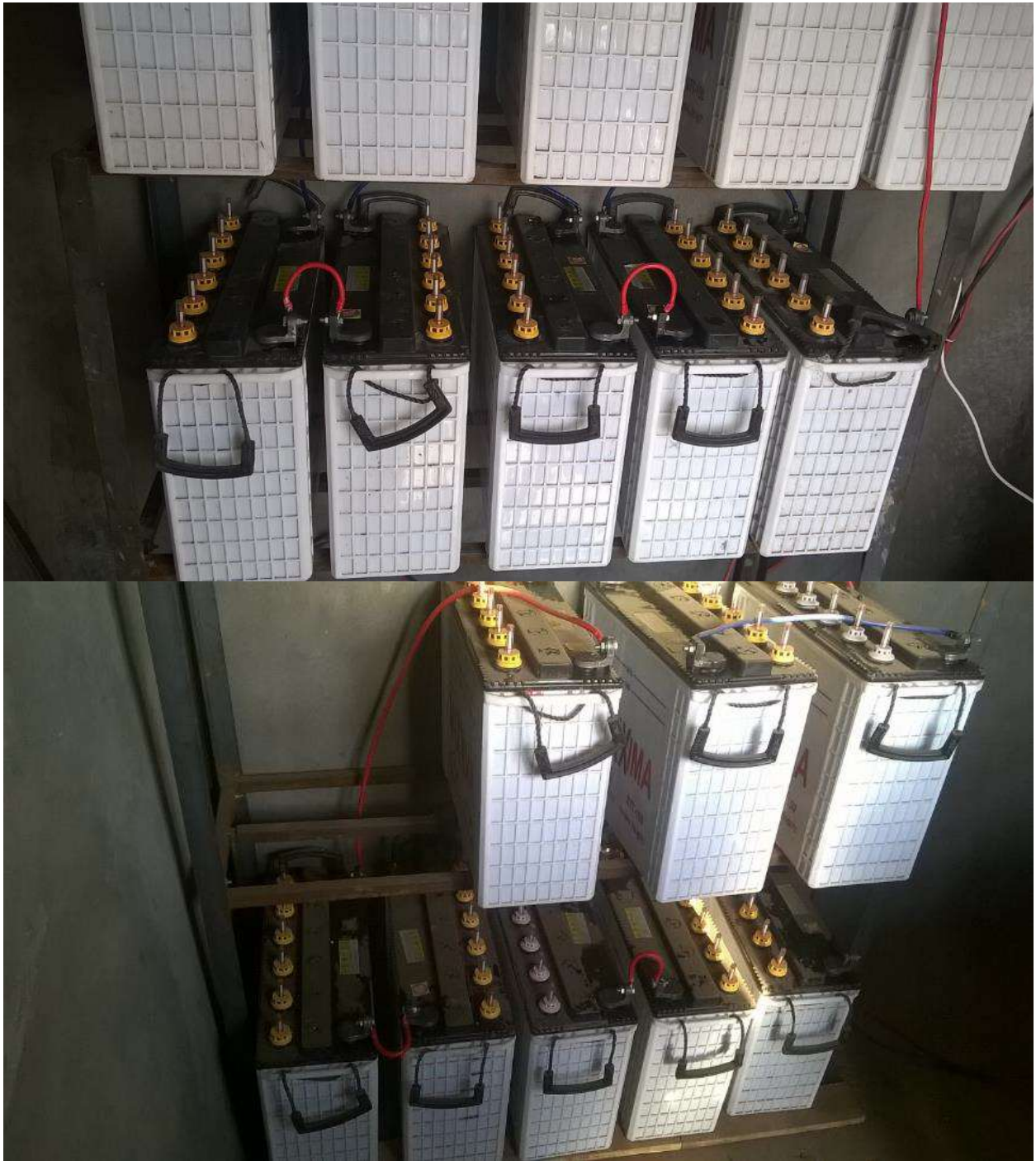
Figure 34 - Batteries housed inside the enclosure control room
