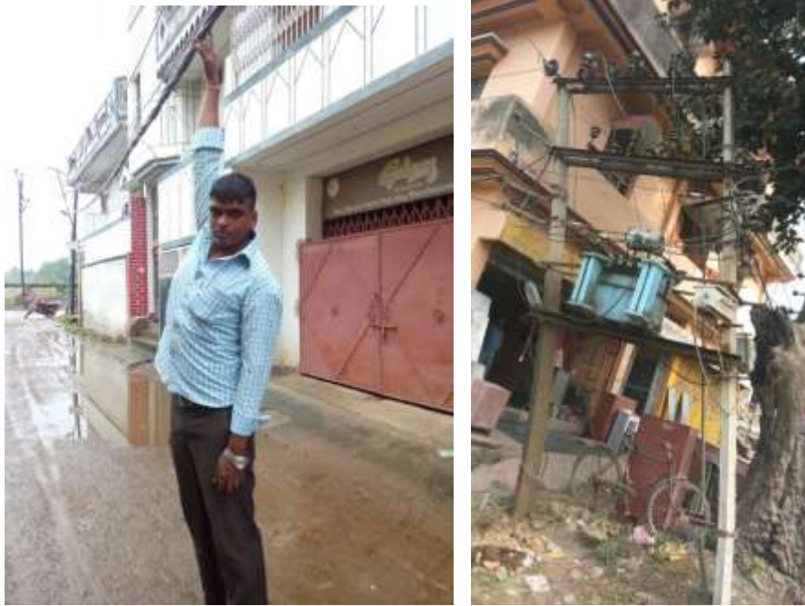
Figure 28 - Low hanging AB cables (left); Disoriented distribution transformer in Bihar (right)
