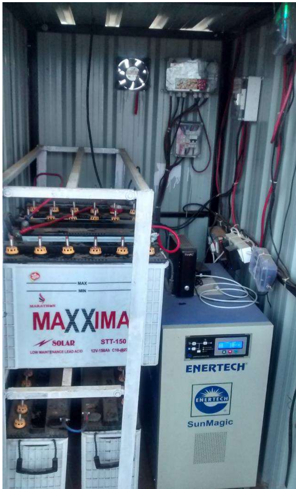
Figure 33 - Inverter housed inside the enclosure
