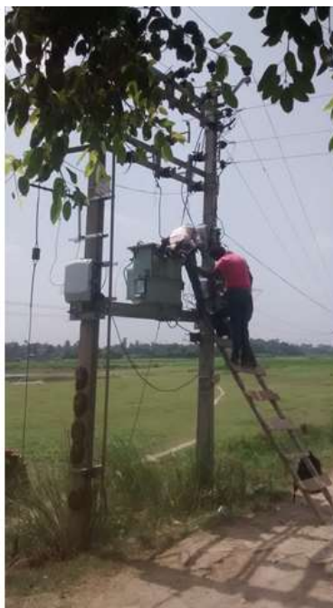
Figure 19 - Images from the installation of Smart meters for grid-connected households
