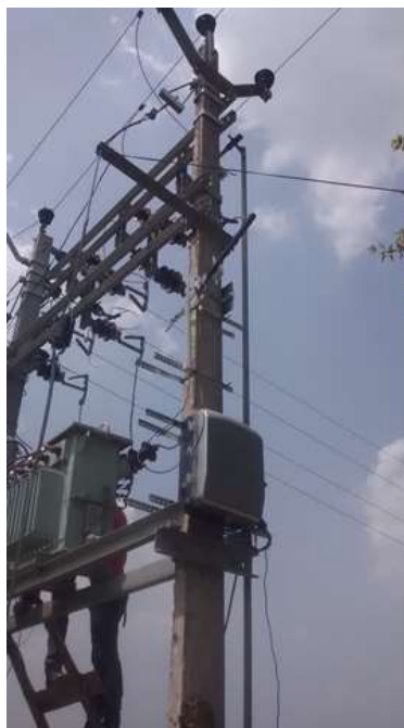
Figure 19 - Images from the installation of Smart meters for grid-connected households
