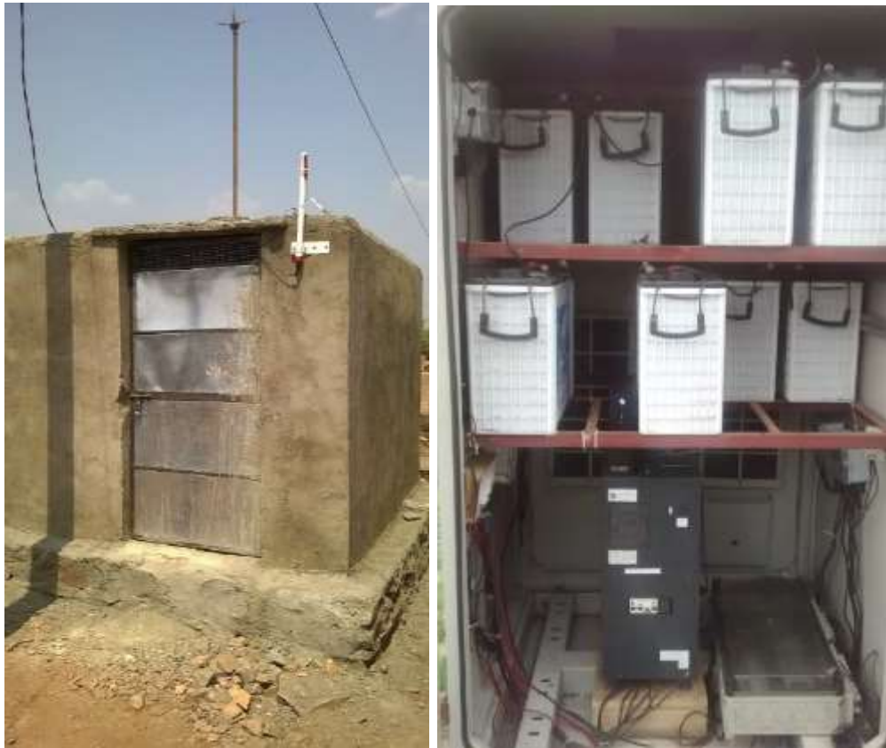
Figure 30 - Enclosures and battery racks
